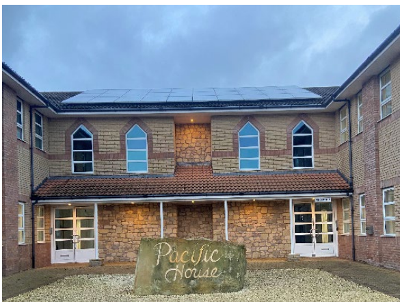
Pacific House, Cumbria Drive Mobility, Carlisle
