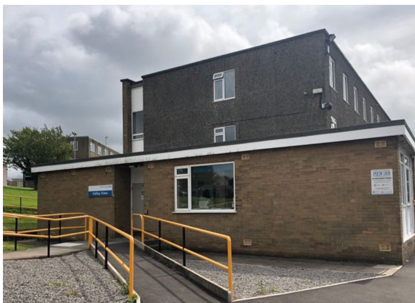
Figure 2 - Valley View at West Cumberland Hospital
