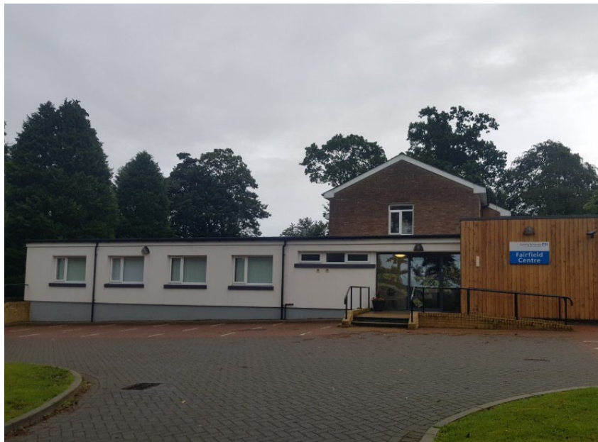
Figure 1 - The Fairfield Centre at Carleton Clinic
